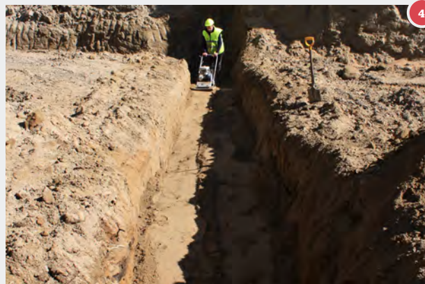
Compacting fill around and over the culvert.
