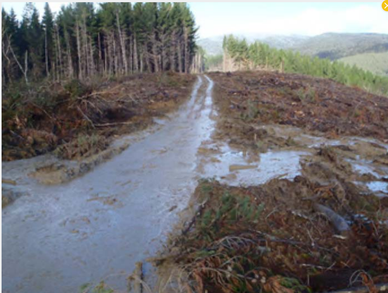
Poorly maintained track – lacking stormwater controls.
