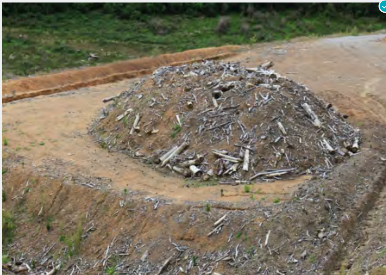
Rehabilitated landing – slash stored in a safe location and water controls installed.
