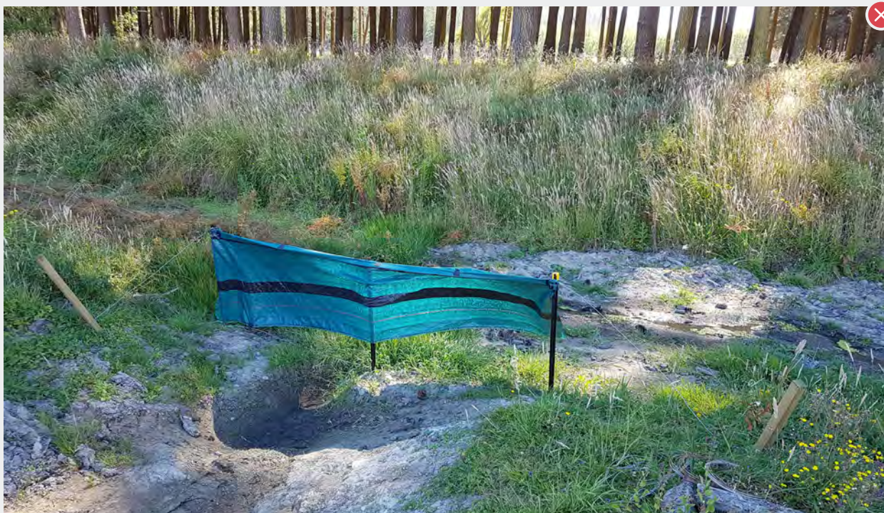
Poorly constructed silt fence.
