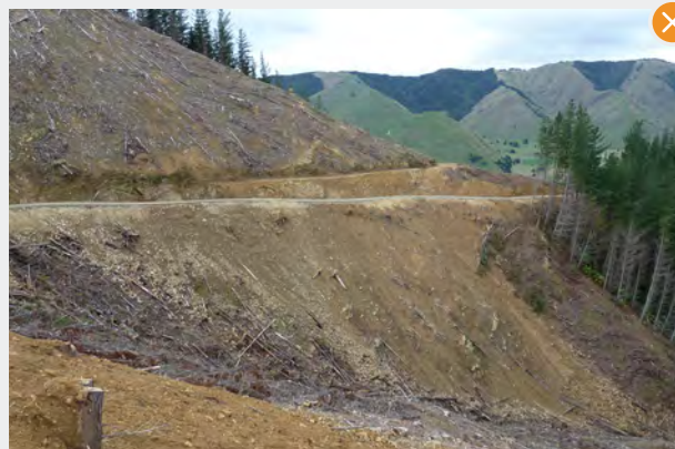
Poor construction practice. The fill material has not been contained and has spilled up to 60 m down the slope. End haul construction should have been carried out to remove spoil.
