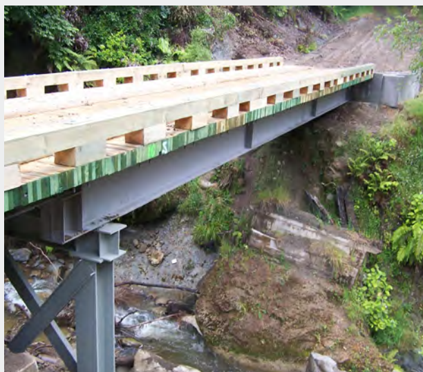
Examples of single span bridges using structural steel and reinforced concrete.
