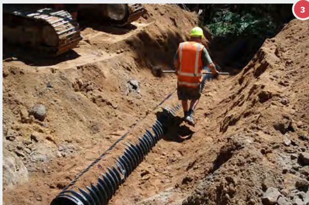
Bedding in the culvert.
