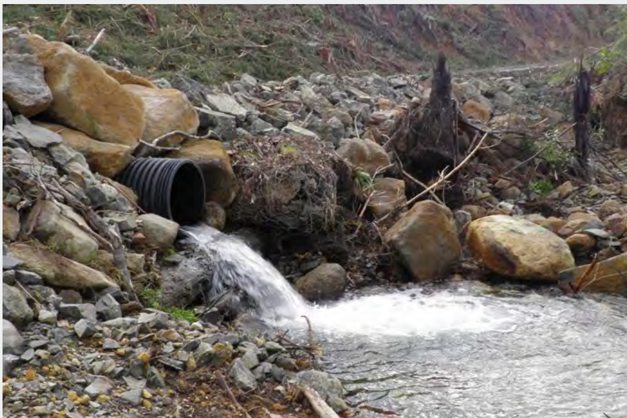
Perched culverts do not allow for fish passage.
