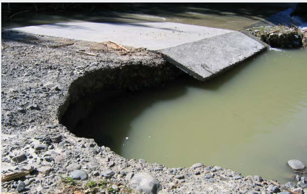
An example of a concrete pad crossing which will minimise sediment mobilisation caused by vehicle crossings.
