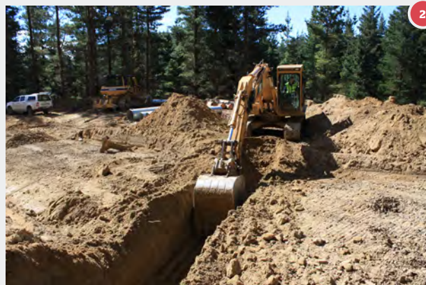
Digging the trench at an angle to the road.
