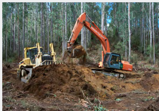
Excavator and bull dozer clearing stumps and stripping prior to bulk earthworks.
