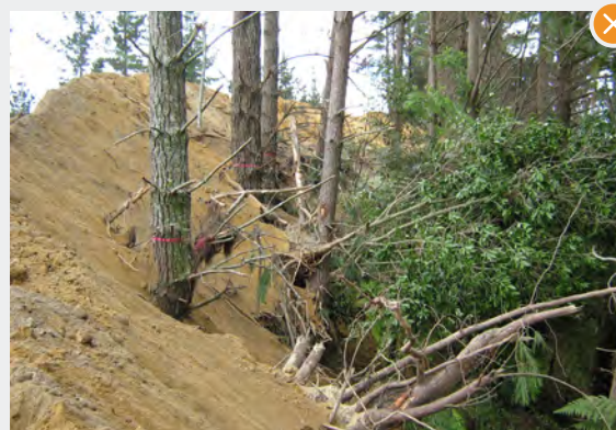
Example of poor road-line salvage where adequate allowance has not been made for road formation and fill has been run into standing trees.
