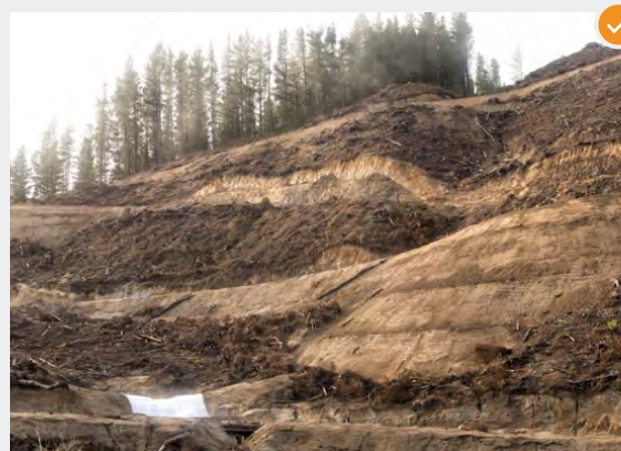
An example of a well-constructed fill batter slope, note flumes controlling the discharge of stormwater run-off and downstream sediment retention pond.
