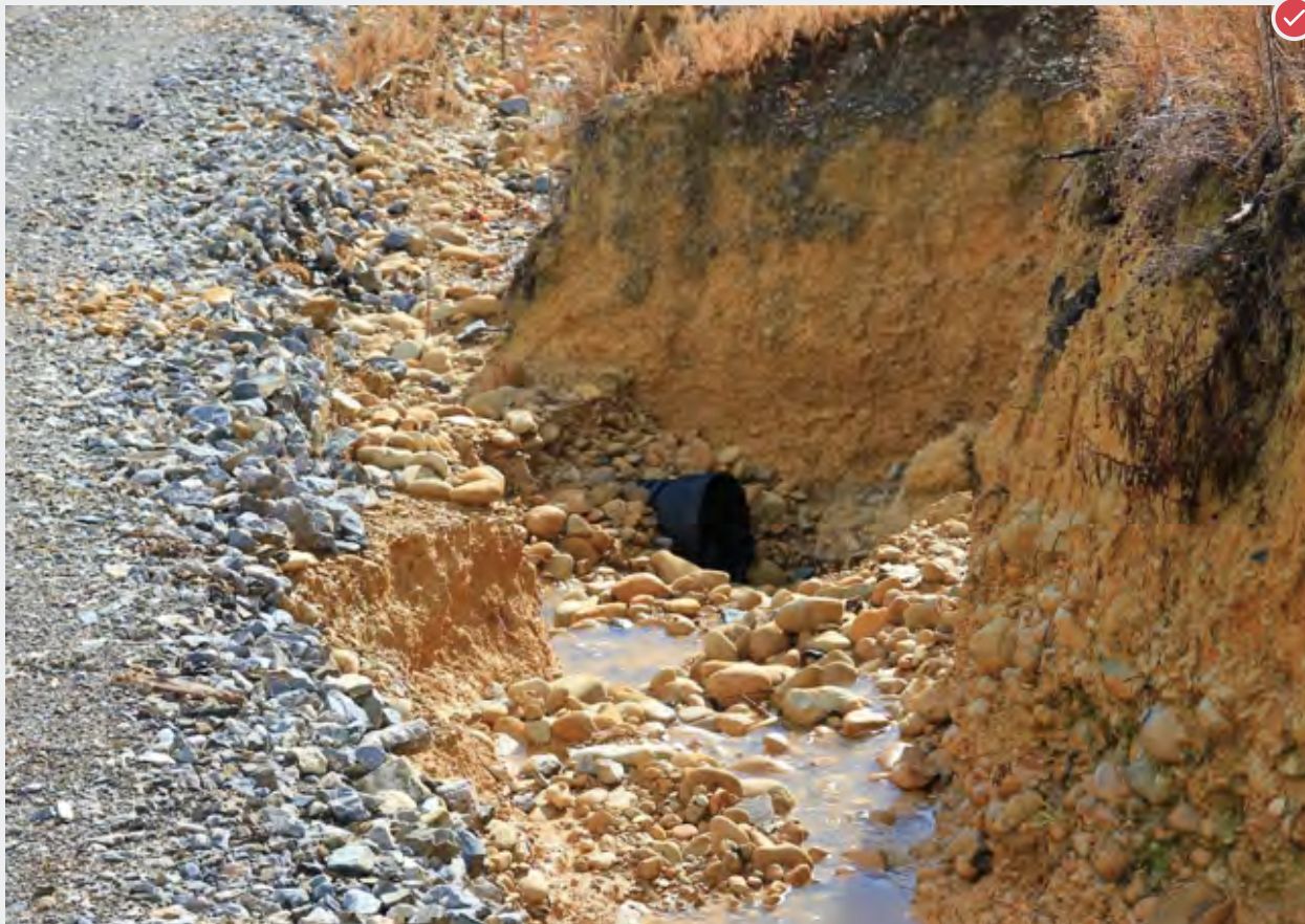
Culvert inlet with batter cut back to allow for maintenance.
