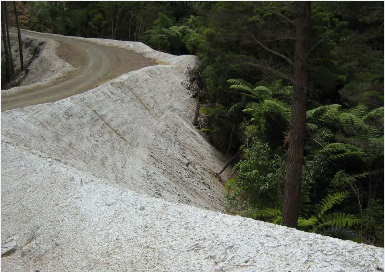
A recently hydro-seeded fill slope.
