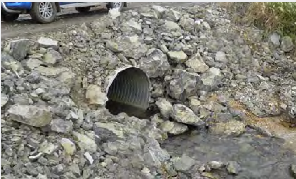
Culvert installation.
