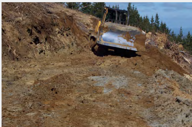
Dozer constructing a pilot roadway.
