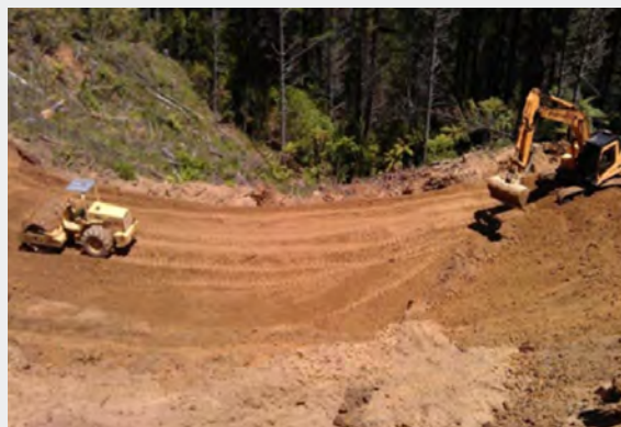
Compaction of a large embankment fill in shallow lifts using a pad foot roller.
