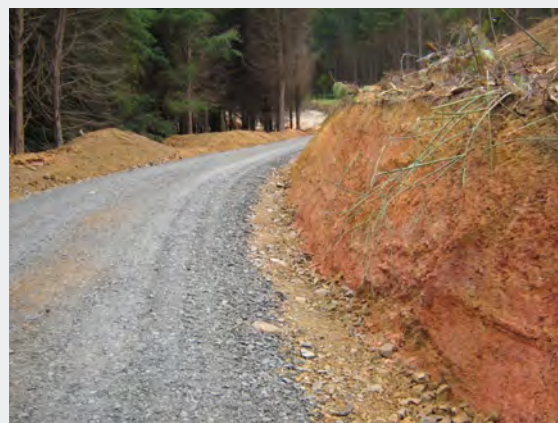
Water table with road base course used for rock armouring.
