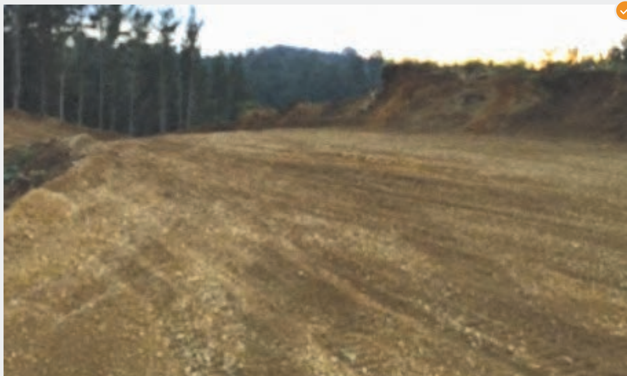
Skid site constructed of a well graded granular fill material – note the range of particle sizes.
