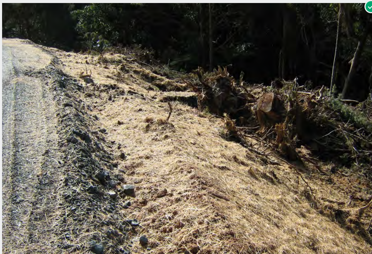
Mulch applied to a road edge providing protection and support for grass seeding.
