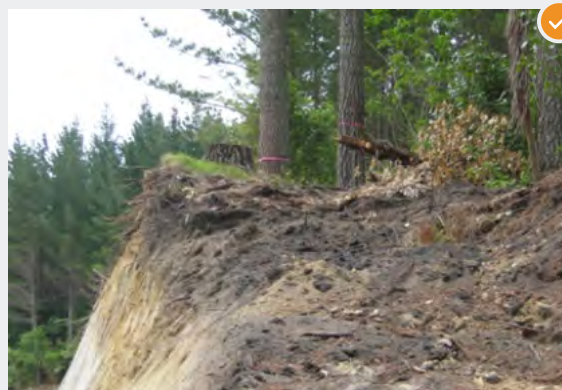
Example of good road-line salvage with a sufficient number of trees removed providing adequate width for road formation.
